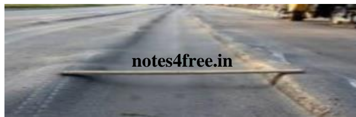
Fig.6: Real-Time Formation of Ruts
